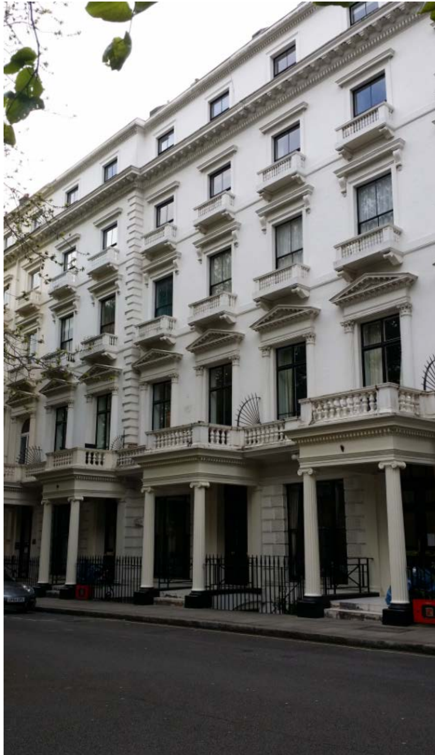
Front Elevation of Application Site
