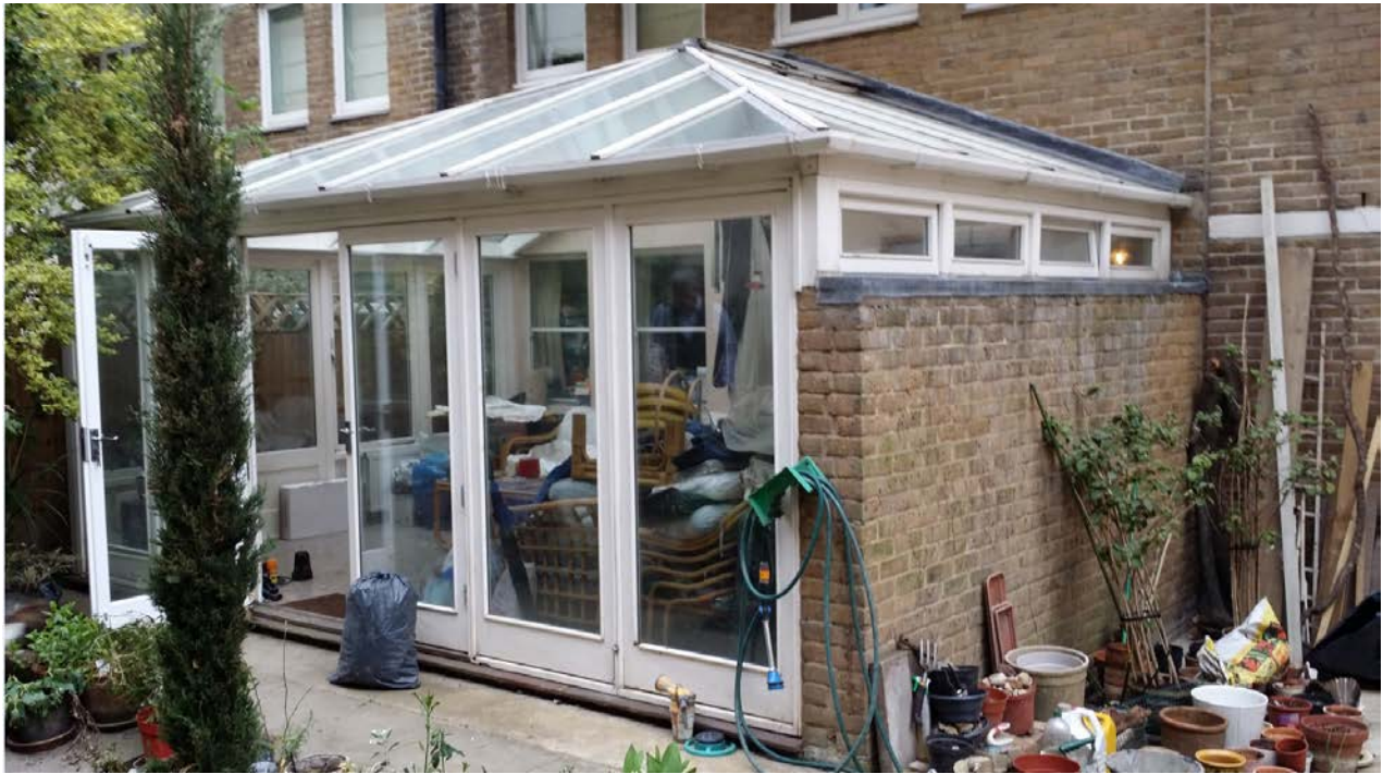
Existing Rear Conservatory
